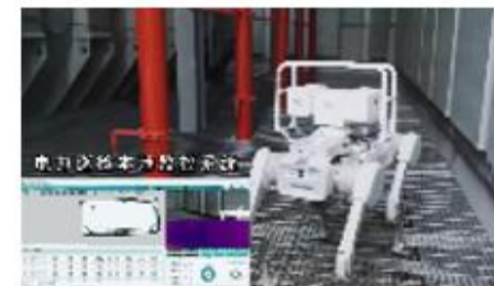
Converter Station Inspection in Zhejiang
